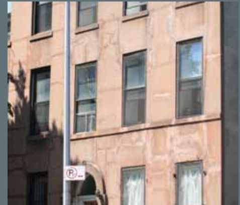
Tinted stucco is an appropriate substitute for brownstone, which is difficult to replace in-kind. However, if possible, it is best to apply stucco in patches to deteriorated areas and not to the whole façade. The rowhouse pictured above has had stucco applied to its entire facade. The coating has cracked in many places, likely due to poor installation, and now water can infiltrate the wall.
