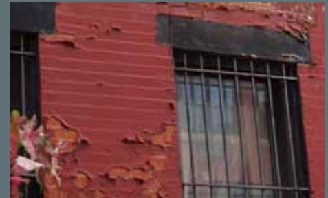
An unnecessary coating of paint on a masonry facade is peeling.
