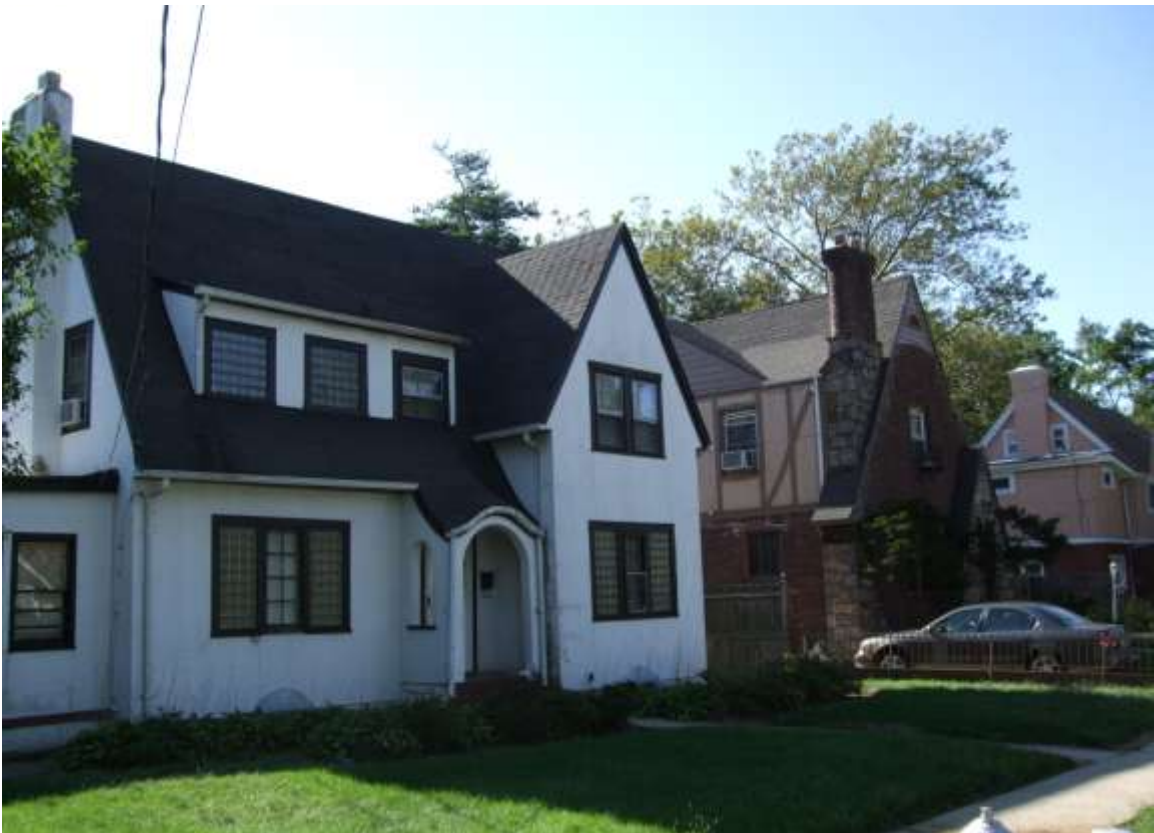
Streetscape #26 West side of 177 th Street between Linden Boulevard and Murdock Avenue Photo taken: September 2008
