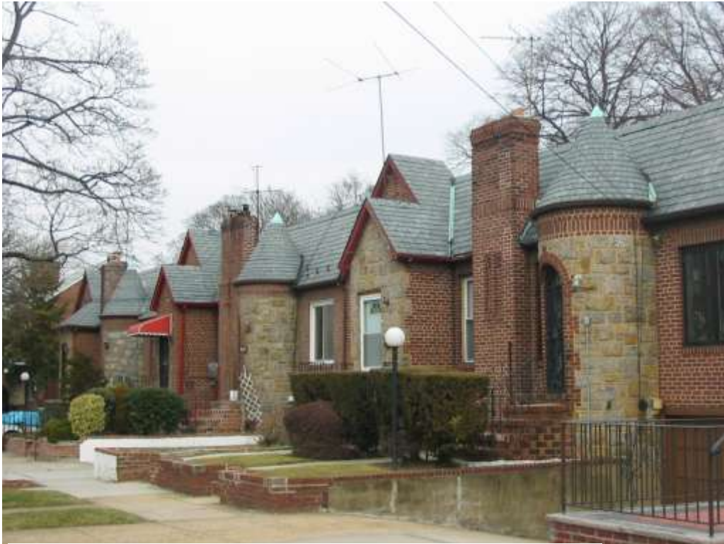
Streetscape #2 East side of 180 th Street between Murdock Avenue & 114 th Road Photo taken: February 2007
