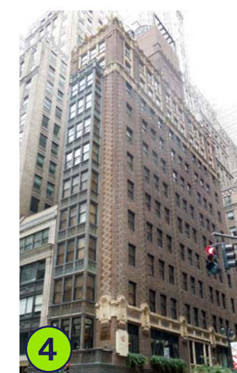
4 299 Madison Ave. Hill & Stout, 1912-13 Built FAR: 13.18 (21.6)
