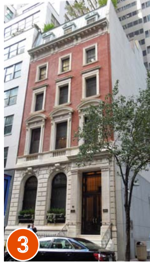
3 39 E 51st St. York & Sawyer, 1902-3 Built FAR: 3.64 (14.4)
