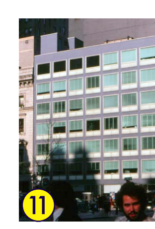
11 532 Madison Ave. Horace Ginsberg & Associates, 1957-58 Built FAR: 8.17 (18.0)
