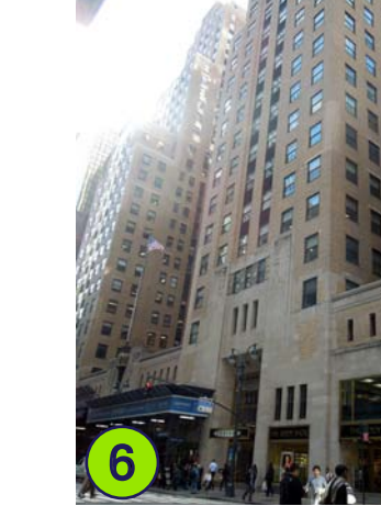
6 Graybar Building 420 Lexington Ave. Sloan & Robertson, 1927 Built FAR: 18.2 (24.0)
