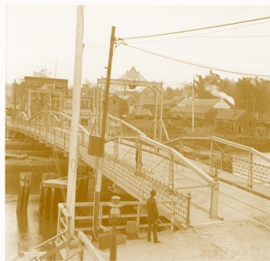
The first road crossing drawbridge at what is now Northern Boulevard.
