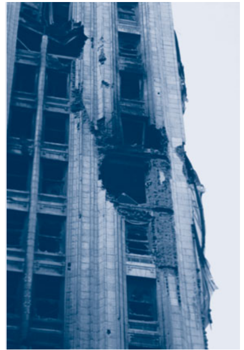
Major hit by steel from the south tower damaged or destroyed terra-cotta and spandrel beams, leaving much masonry unsupported.
