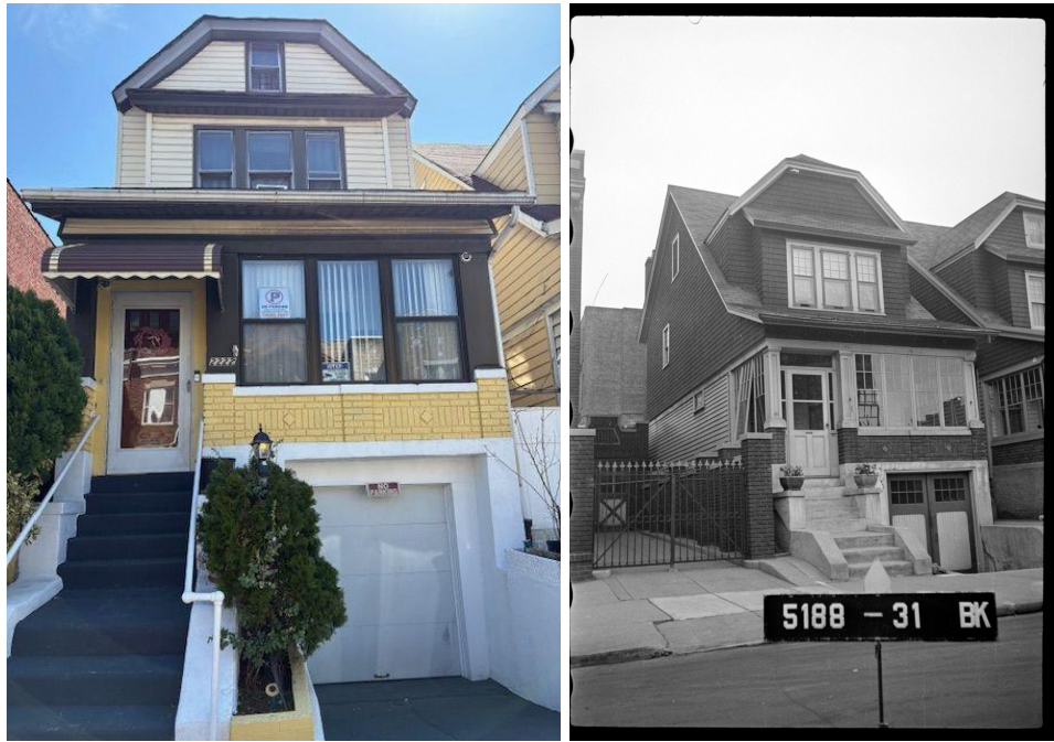
2222 Vanderveer Place, current condition (Left) and 1940's Tax Photo (Right).
