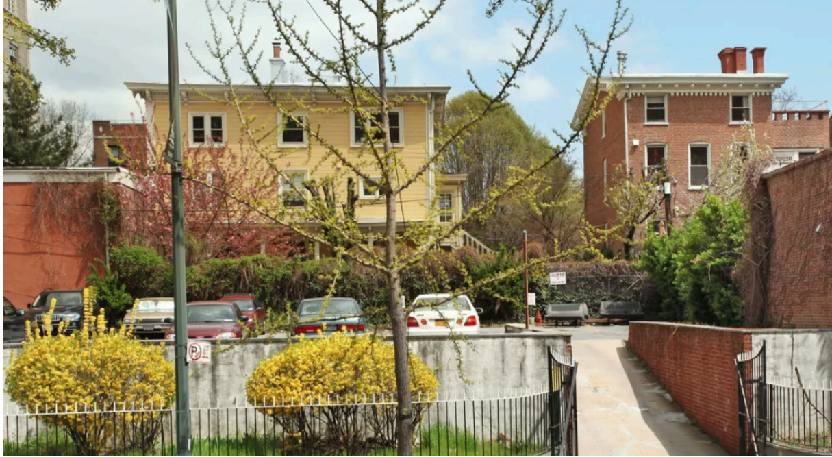
Back of the house showing window configuration and back porch (Source: Corcoran)
