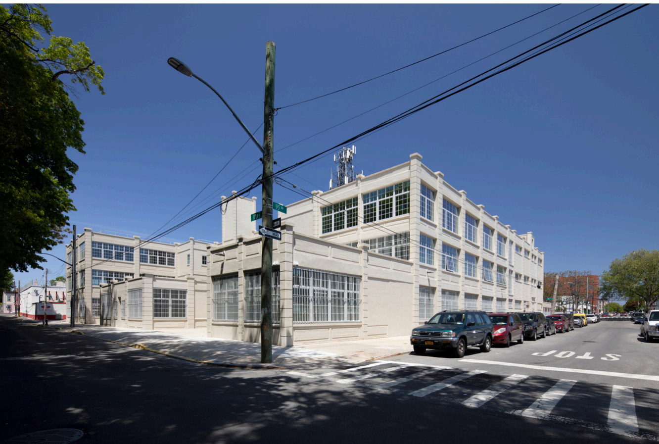
Exterior views of GMDC's rehabilitation of a 1906 factory building in Ozone Park . Using historic rehabilitation tax credits, the project preserved the building's industrial infrastructure while adapting it to accommodate 23 contemporary manufacturing businesses. Top photo: Tim Soter. Bottom photo: © Frederick Charles.
